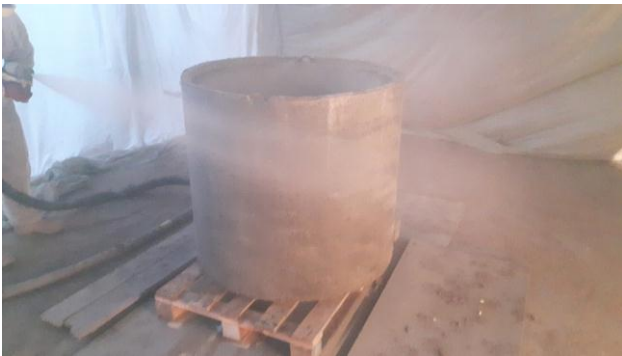
Fig. 5 Spraying polyurea coating system on concrete ring
